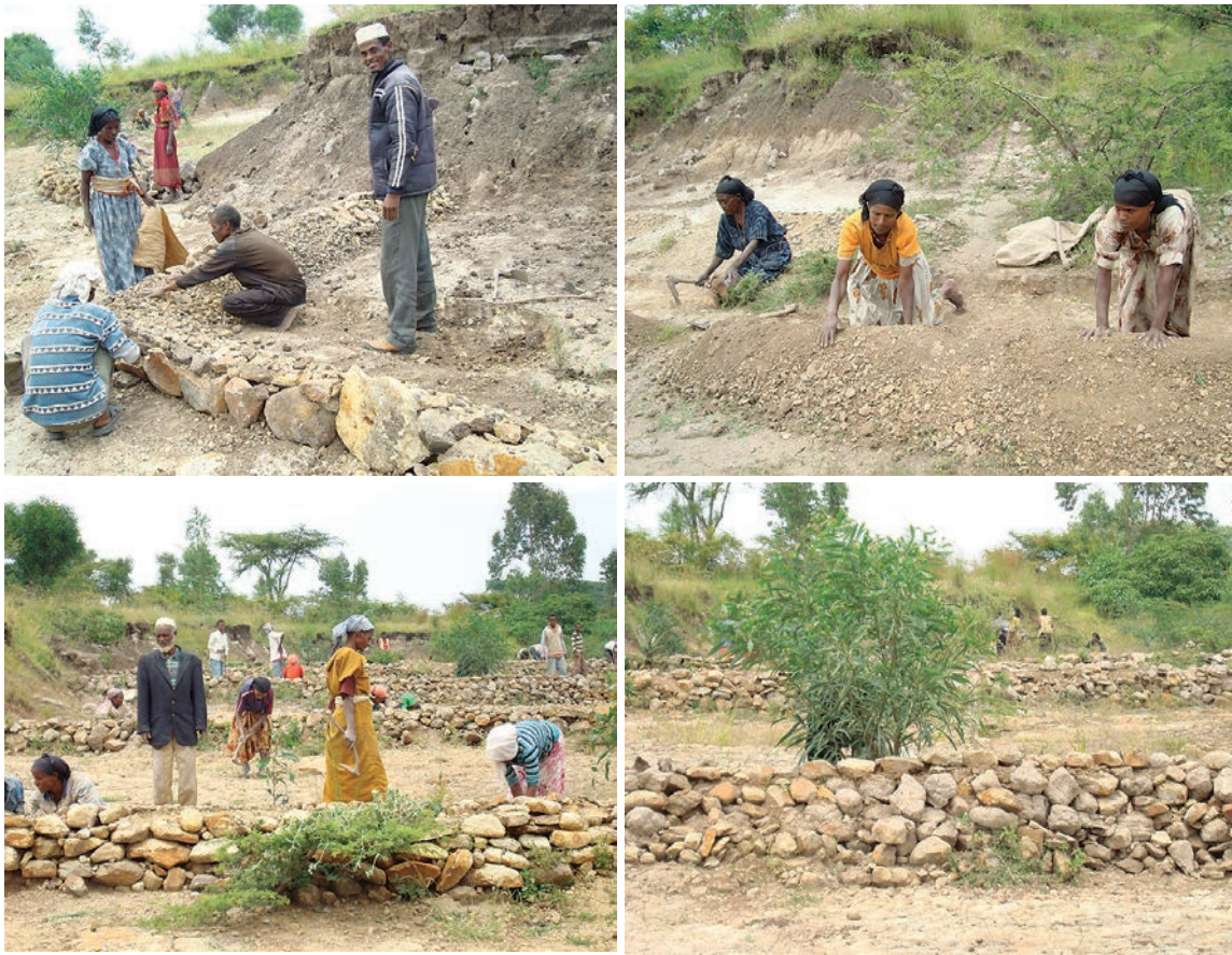
Figure II 18.3 Local people constructing physical soil conservation structures and planting trees and grasses on degraded land at Choroko, Alaba, southern Ethiopia. ©Alaba Agricultural office
