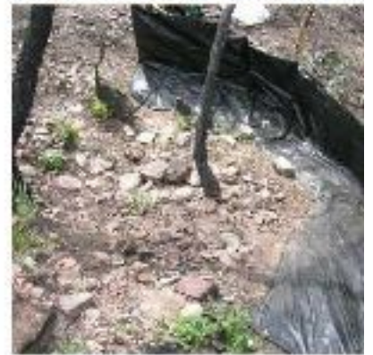
Silt-fence used to monitor sedi
